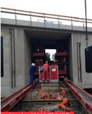
Kreuzungsbauwerk Hafenbahn KEG - Krefeld, Di Item details: Rail bridge of 950 ton Equipment: Sliding system and gantry crane
